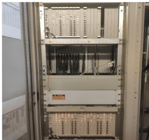
Figura 16 - Interfaces DCS (Navigator Pulp Aveiro, 2023).
