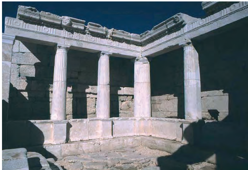
Figure 4 - General view after the restoration works, September 1997.
