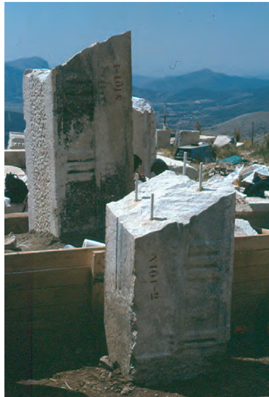
Figure 9 – For joining the architraves, fibreglass rods were used together with the epoxy adhesive.
