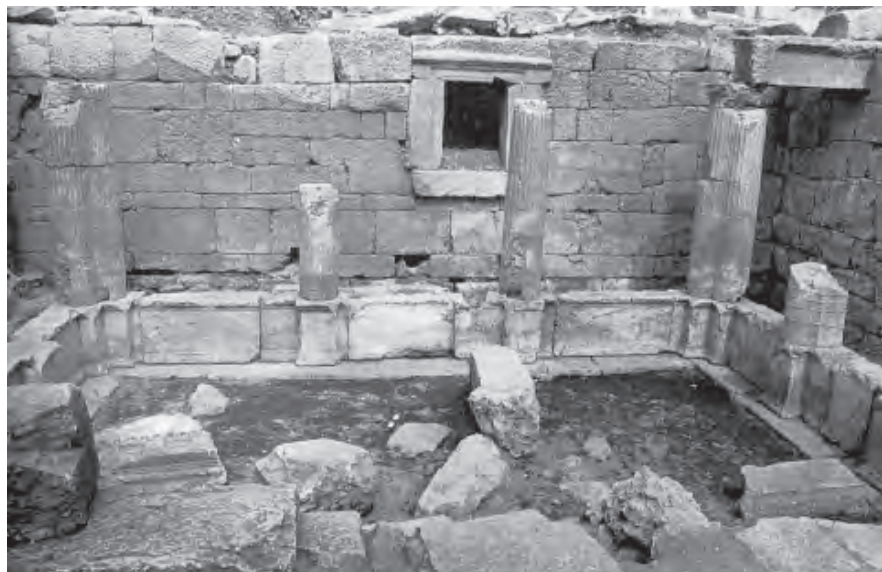
Figure 3 - General view before the restoration works, August 1993.
