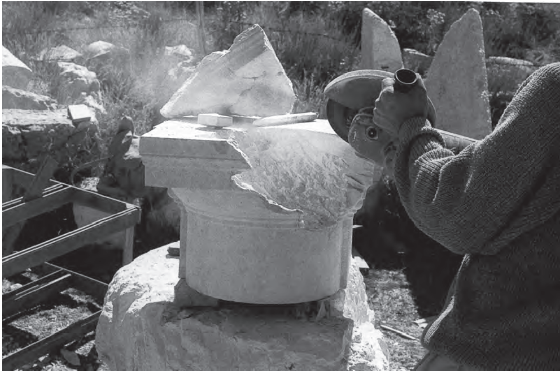
Figure 13 – Preparing a new carved capital for the insertion of the existing fragments from the original capital.
