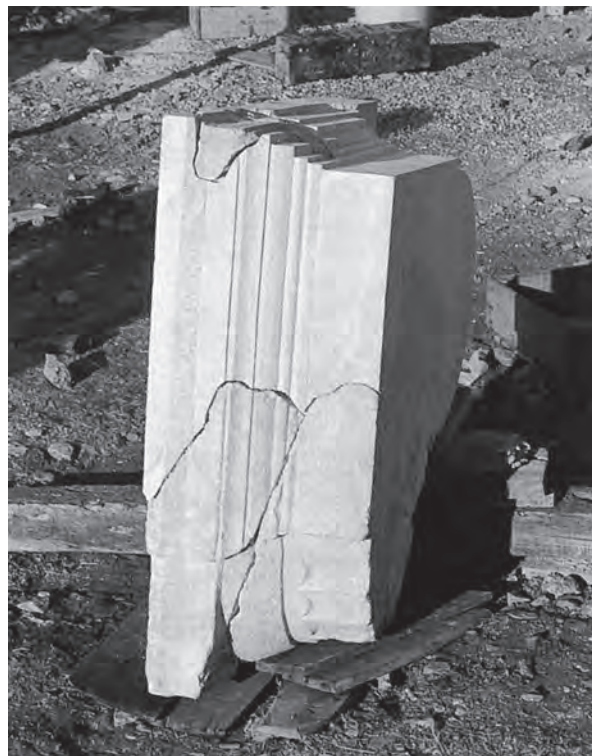
Figure 14 – Insertion of original fragments in a new carved capital.
