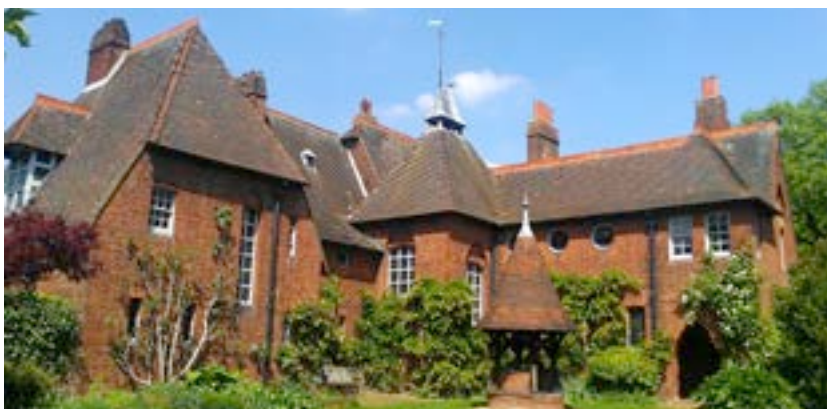
Ilustração 2 - The Red House: fachada lateral, William Morris, Philip Webb e Burnes-Jones. (Unthank, 2016).
